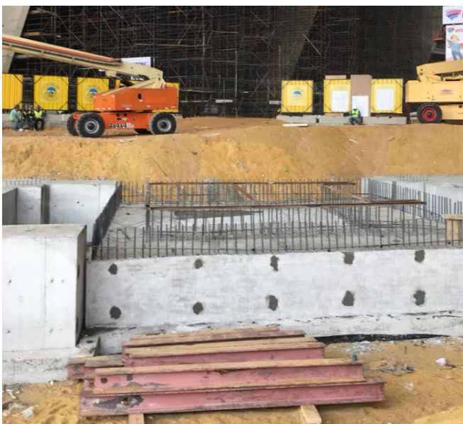
Xypex treated concrete base.
